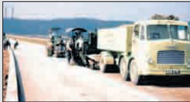
● THE road construction included a layer of a material called "wet mix". This picture shows the material being laid and rolled.
